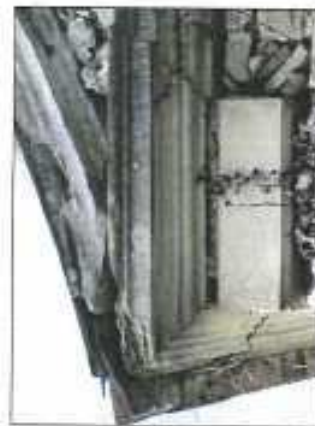
Corniche fronton Angle S-O
